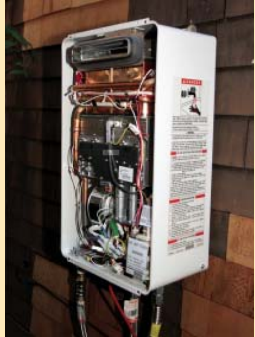
Figure 2. This on-demand gas heater (shown without its cover) has sophisticated controls to regulate the burner and combustion fan based on flow rate and incoming water temperature. It has more in common with a high-efficiency furnace than with a conventional water heater.
